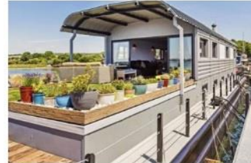
Energy Management: the MAC1010 floating sustainability project
